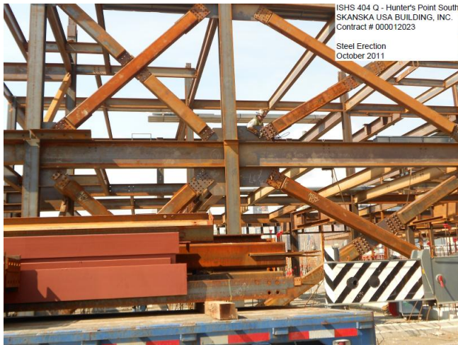
Figure 17: Lateral bracing erected
