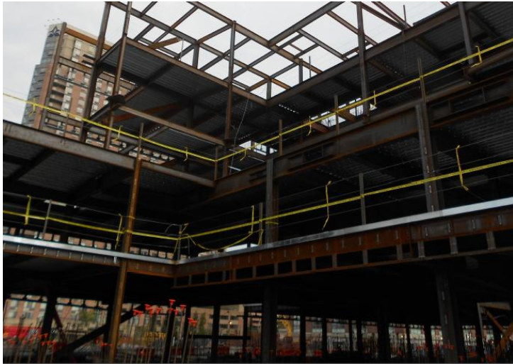
Figure 14: Steel Frame Erection Photo by SKANSKA Inc.
