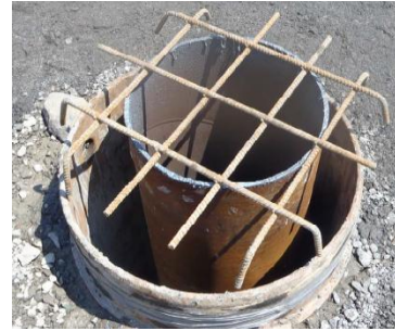
Figure 9: Isolation Casing Photo by SKANSKA Inc.
