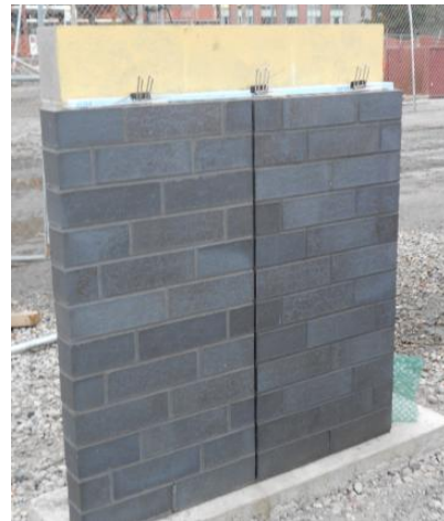
Figure 4: Typical Wall mock-up Photo by SKANSKA Inc.
